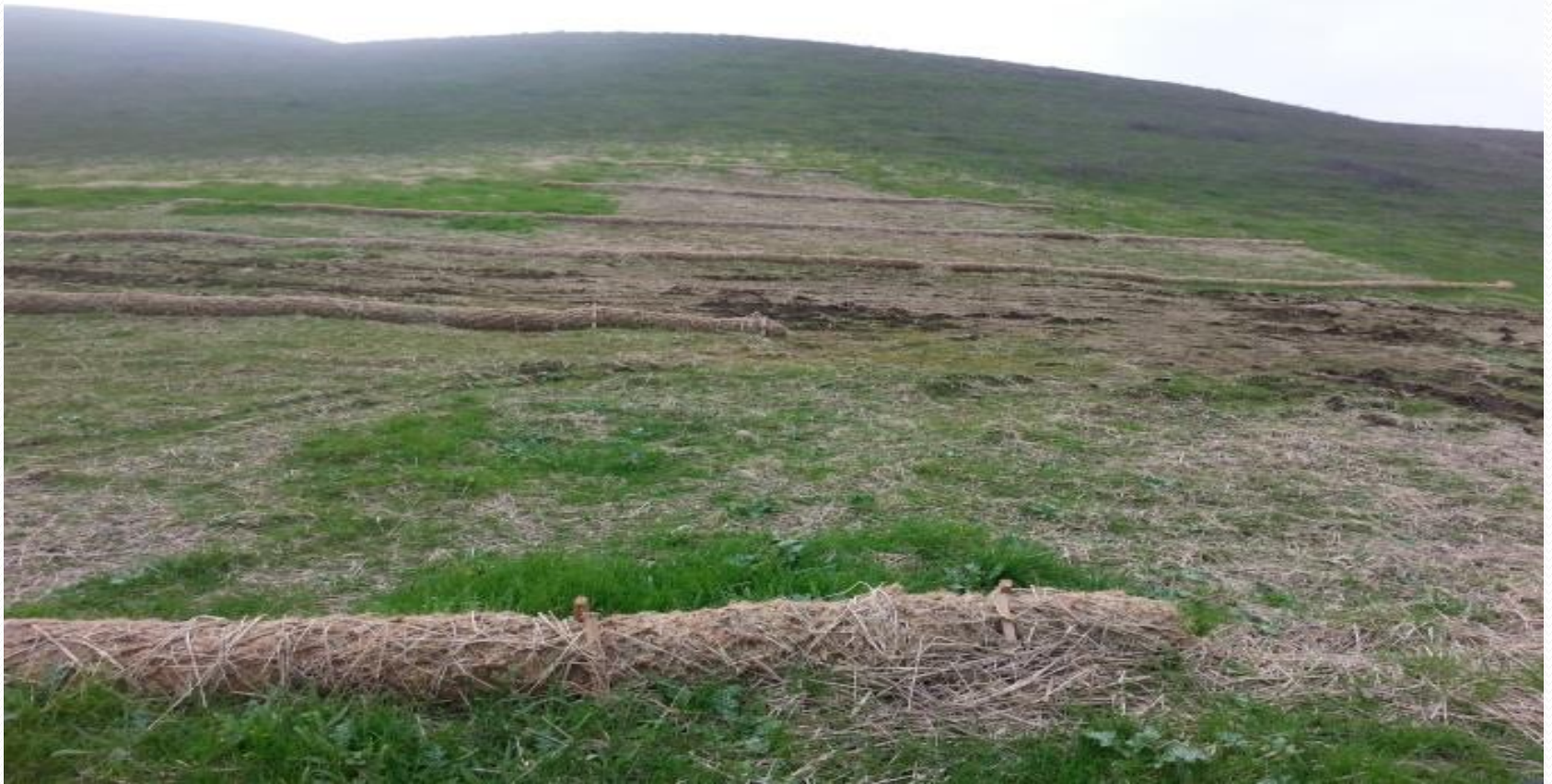
Pit 1, backfilled, reseeded, and staked with coir rolls
